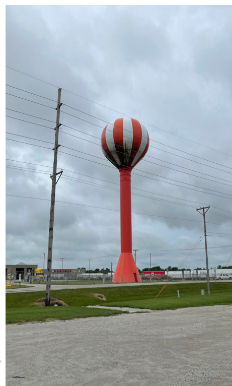
Figure 8.1 – Water Tower and Utility Lines
